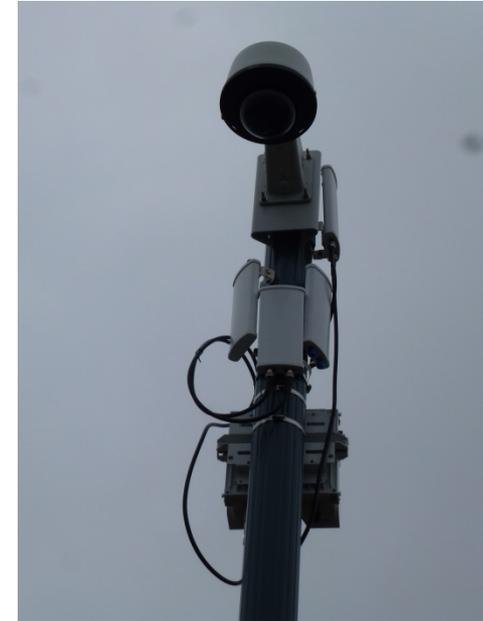
Antennas should not be placed directly against walls. This results in adverse changes to the pattern, as well as wasted signal absorbed into the structure.
