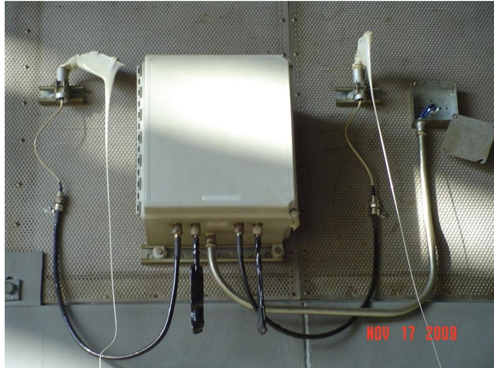
**Do not place antennas and enclosures immediately behind F-18 jet engines!**
