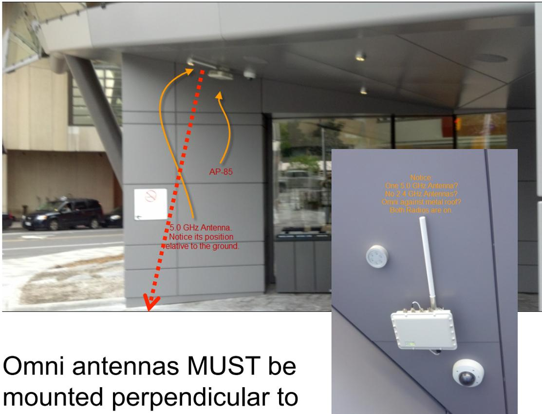
Omni antennas **MUST** be mounted perpendicular to the ground.
