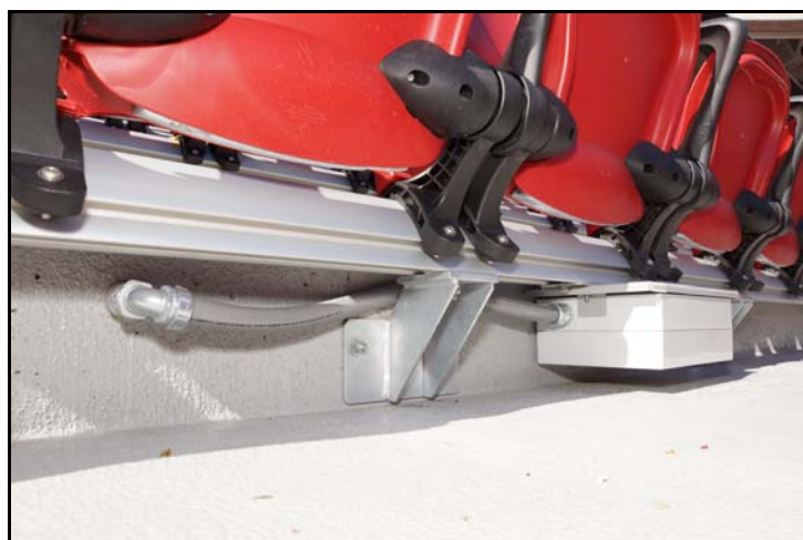
Figure P3-7 Examples of Underseat Picocell Coverage in Stadiums
