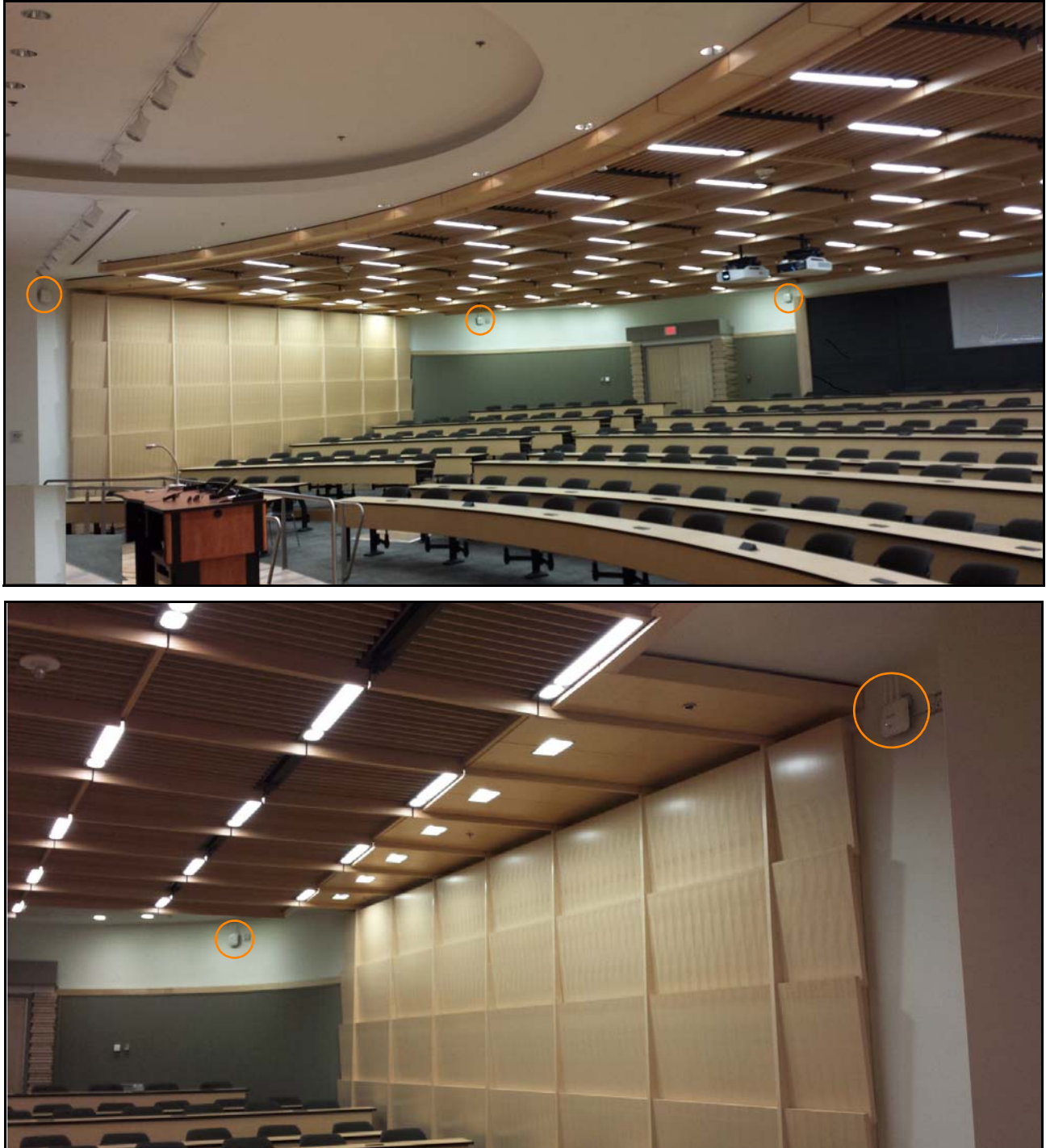
Figure P3-5 Side Coverage Deployment in University Lecture Hall
