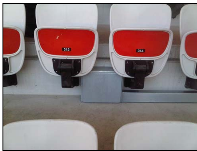
Figure P3-7 Examples of Underseat Picocell Coverage in Stadiums
