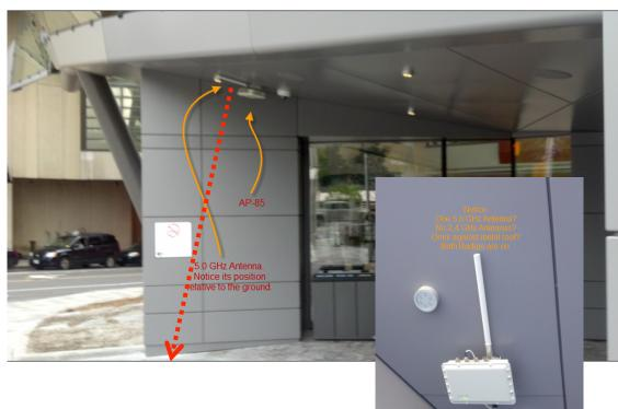
Omni antennas MUST be mounted perpendicular to the ground.
