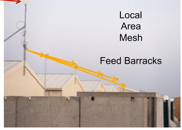
LAM AP's feed 2.4 GHz inside each barrack with Indoor antenna - serves 1 to 20 Users
